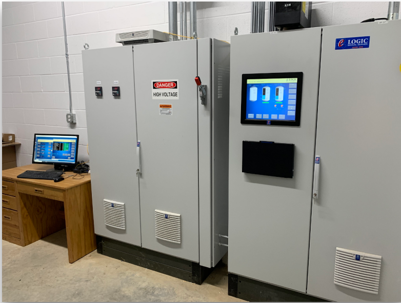
Main SST Controller Cabinet with VFD Cabinet and Remote Workstation
