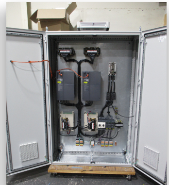
VFD Condenser Panel with Starters for Pumps
